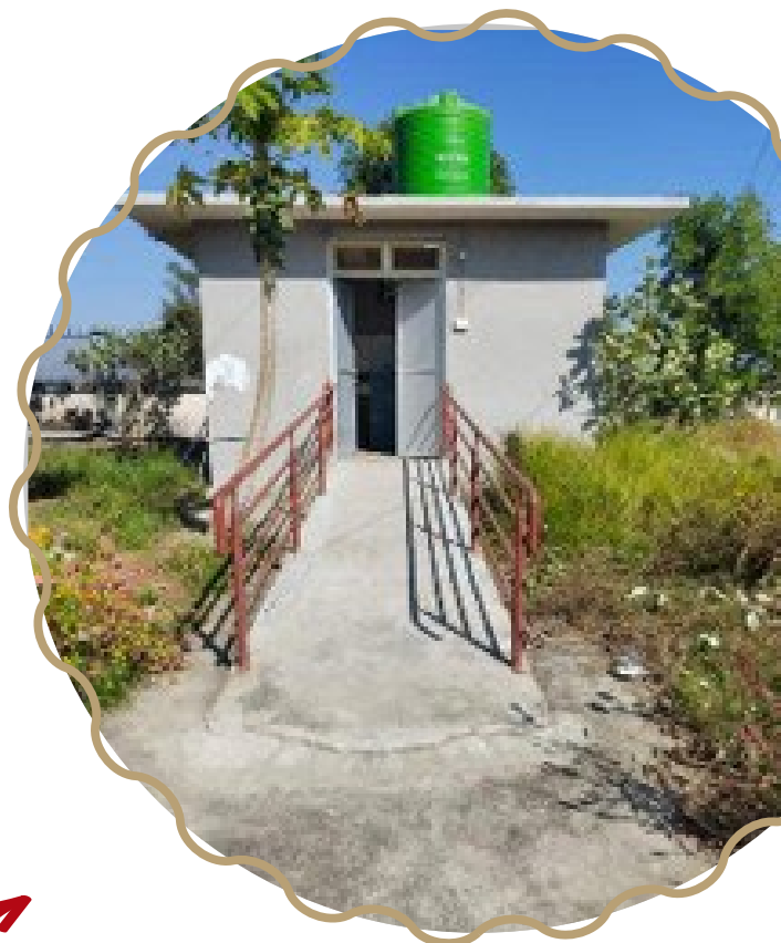
An accessibility ramp providing safer and more inclusive access to toilet facilities at a Provincial Rehabilitation Centre.
